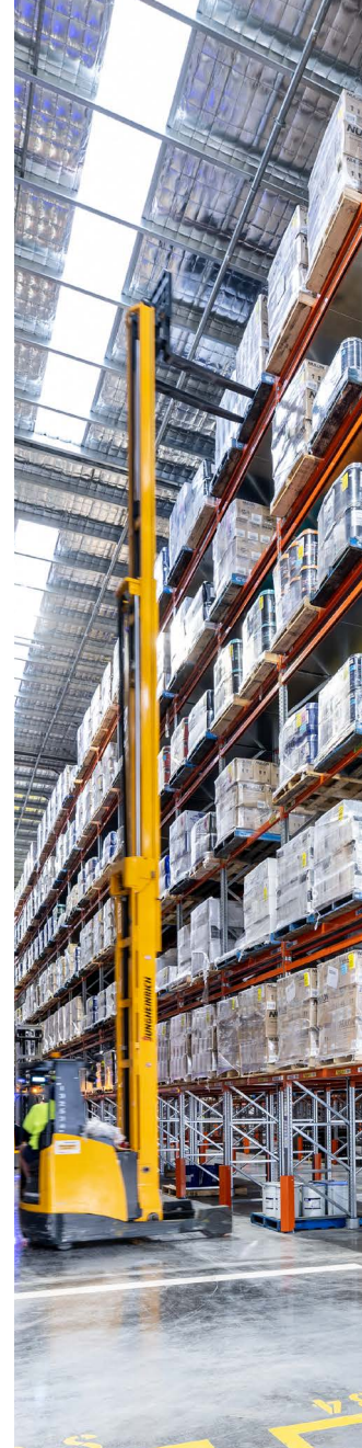
ALIRO CASTRO WAY LOGISTICS FACILITY
